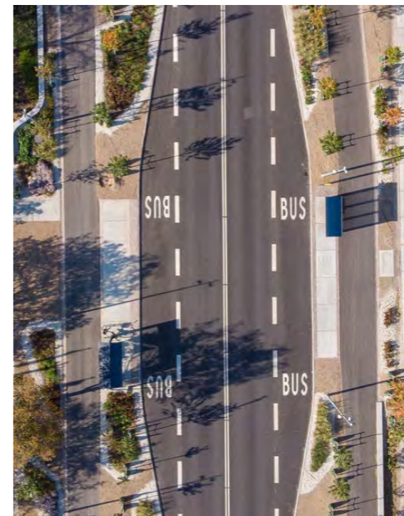
upgraded bus stops
