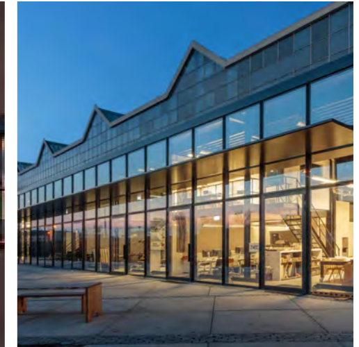
Improving access to natural light
